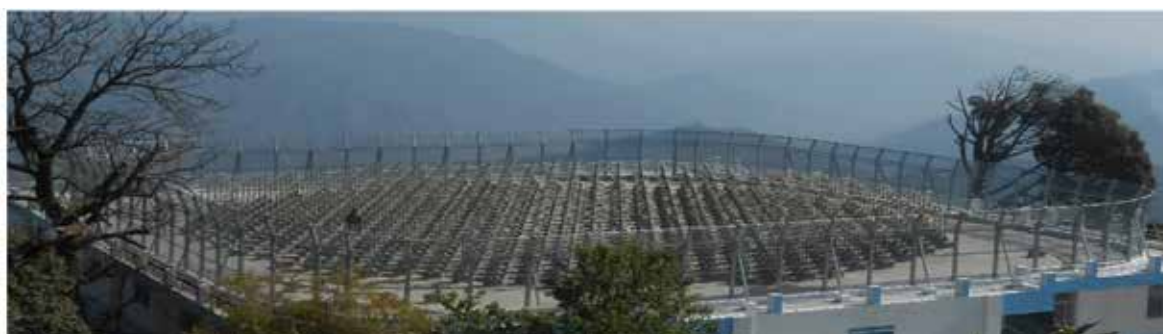
Figure 53. ASTRAD antenna array on the roof-top of the ASTRAD building with recently installed clutter fence along the periphery of the antenna array.
