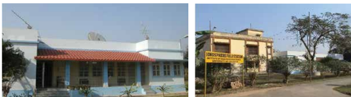
Figure 54. ST Radar System at University of Calcutta, West Bengal.
