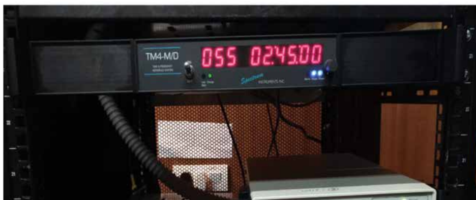
Figure 42. The image shows the GPS receiver and Rubidium clock installed at the ORT. The black panel on the top is the GPS unit (Spectrum TM4M/D) and the bottom right panel shows the Rb clock (FS725).
